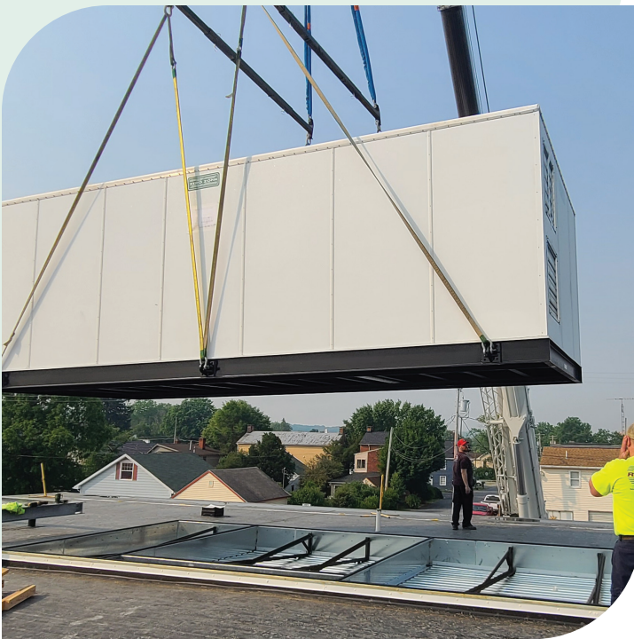
Installation of Custom Electrical Mechanical Center
