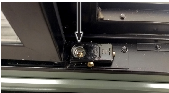
FIGURE 31: Torque Adjuster Locking Screw
