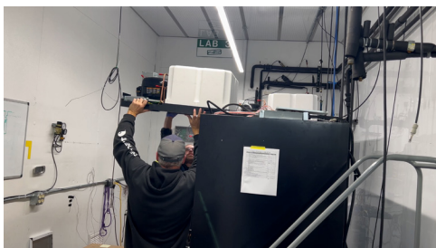
FIGURE 14: Lifting the PRU
