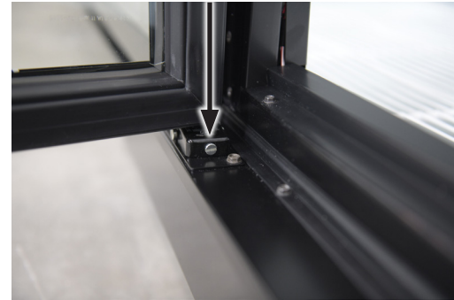
FIGURE 21: Sag Adjustment Screw
