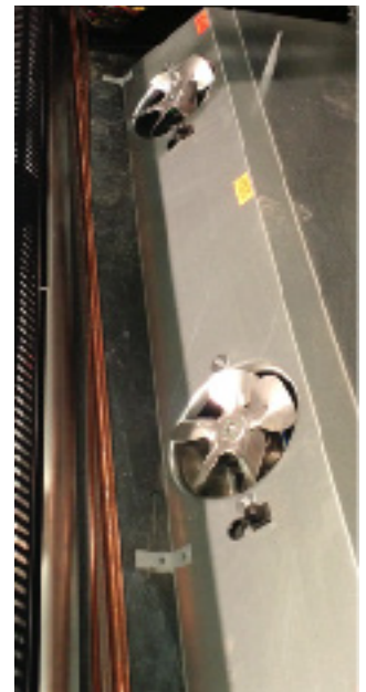
FIGURE 45: Fans and Case-to-Case Piping
