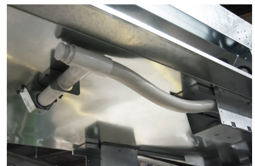
FIGURE 19: Drain Installation
