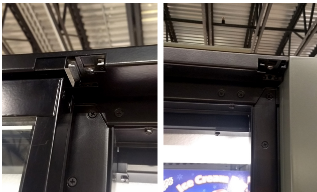
FIGURE 31: Switch the Hinge to the Opposite Side
