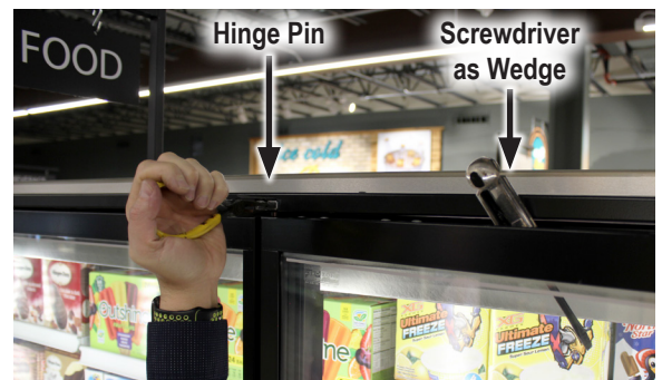
FIGURE 26: Use a Wedge & Pinch Hinge Pin
