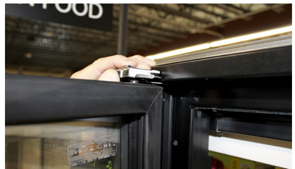
FIGURE 27: Push Door & Hinge Pin into Place
