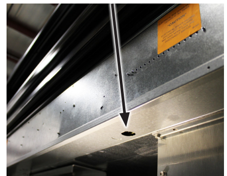
FIGURE 52: Electrical Supply Access Hole
