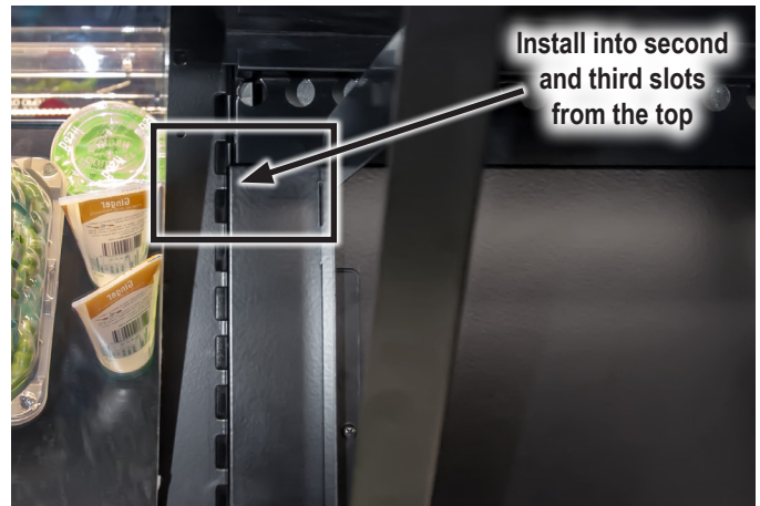
FIGURE 28: Shelf Standard Slots for Air Deflector
