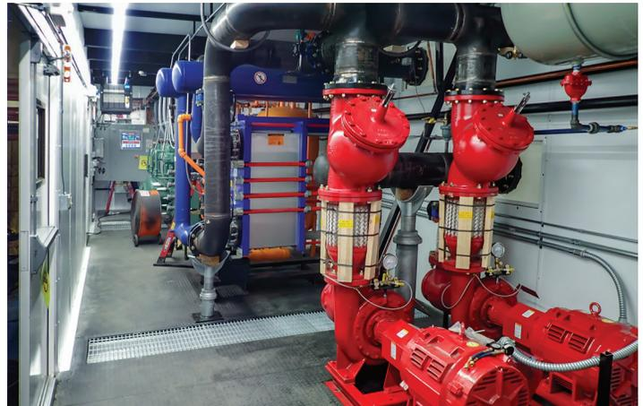
**System 2:** HFC/HFO system with direct expansion plate chiller (**FIGURE 2**).
